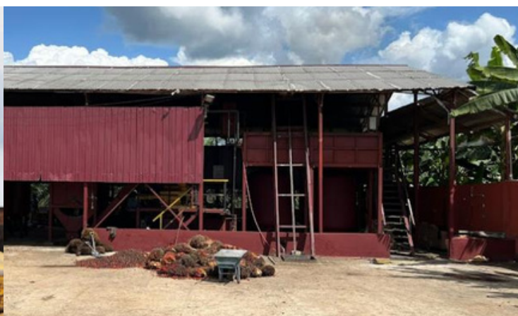
New oil palm processing machinery
